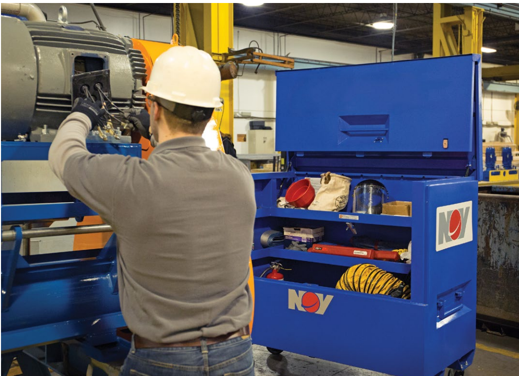
Experienced field service technician repairing equipment on site to minimize downtime
