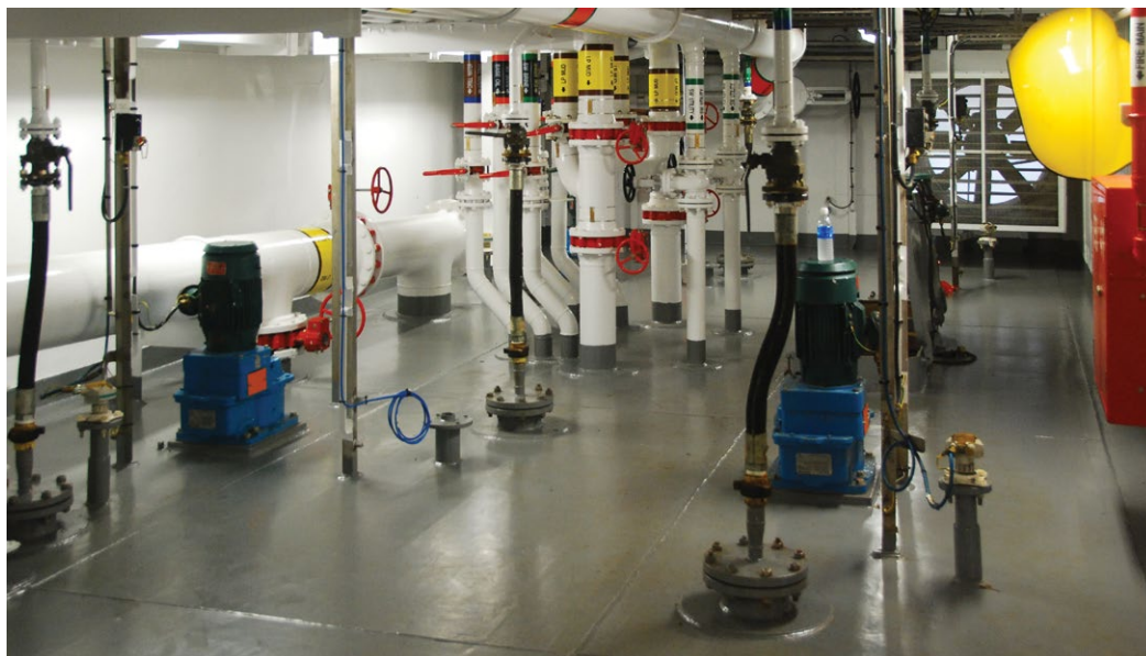
Installed Model 20 agitators on an oil rig
