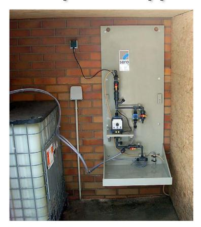
Wastewater treatment plant: CVD1-60.1 with a R204.1 / Medium: Aluminium chloride
