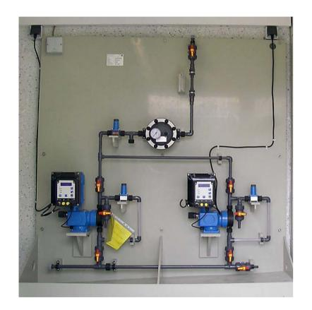
Wastewater treatment plant: CVD2-60.1 with two C409.2 / Medium: Iron(III) Chloride
