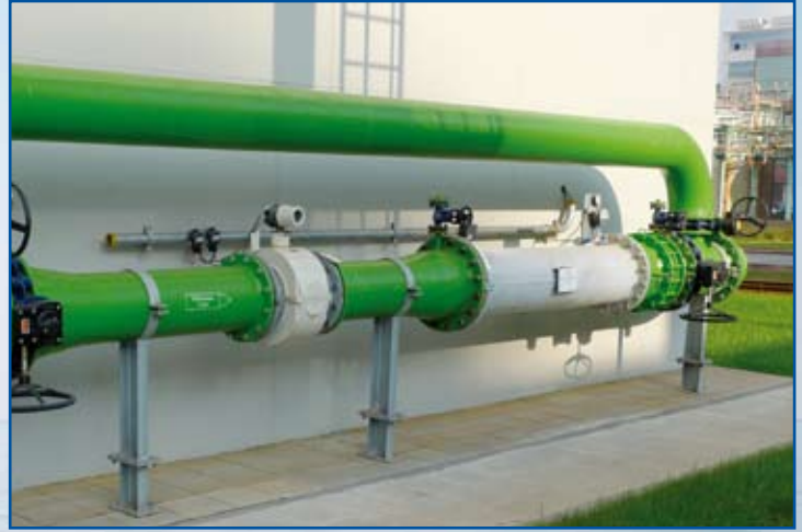
Fig. 9 river water filtration in chemical works
