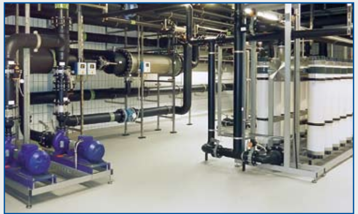
Fig. 11 drinking and process water filtration in brewery
