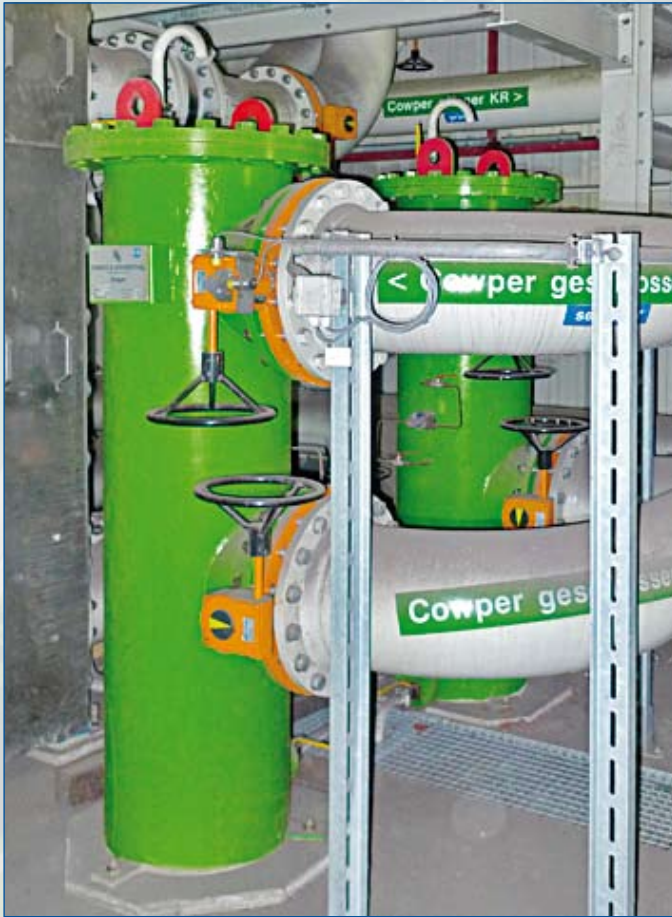
Fig. 2 Single Filter in welded steel design
