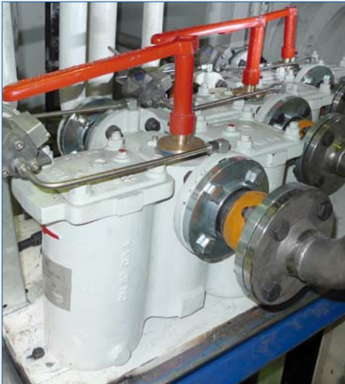
Fig. 4 Duplex Filter in cast iron design
