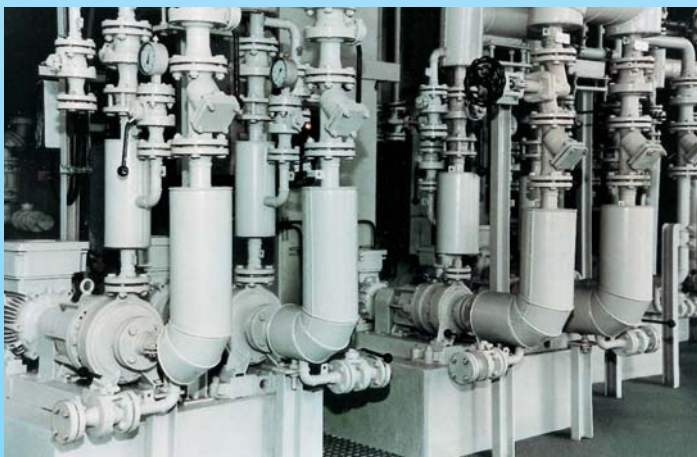
Type NML with magnetic coupling. Liquid: Acetic acid, 130°C (266°F).
