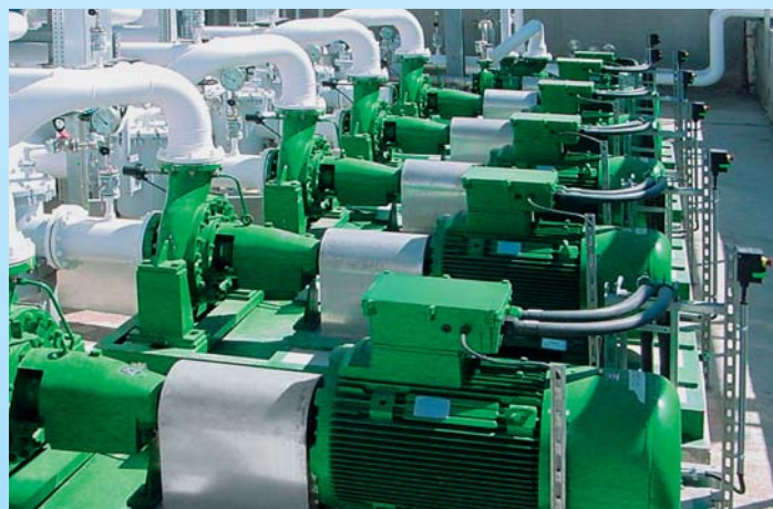
Type NCR – API 610 7th ed. – with single mechanical seal. Liquid: Aviation fuel JP4.
