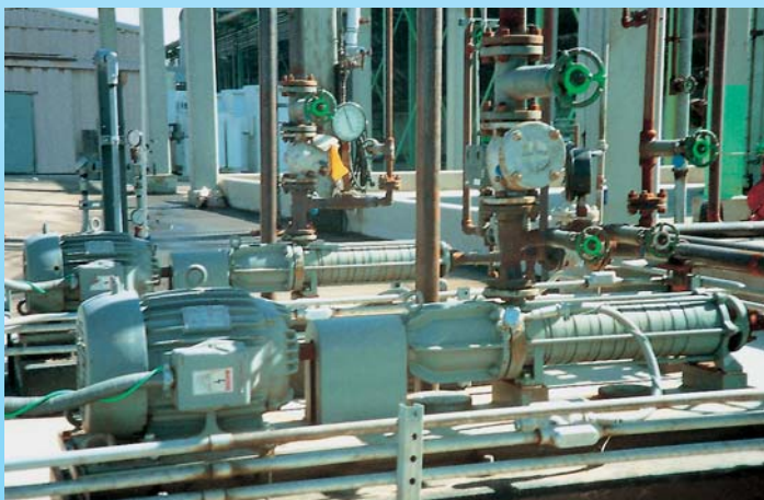
Type SCM with magnetic coupling. Liquid: Methanol, 40°C (104°F).
