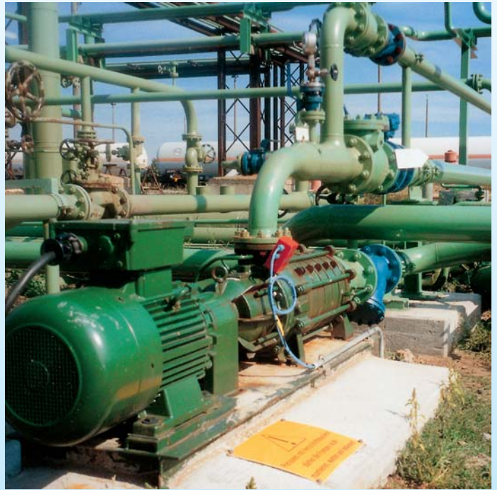
Type HZSMA with magnetic coupling. Liquid: Propane/Butane, 20°C (68°F).
