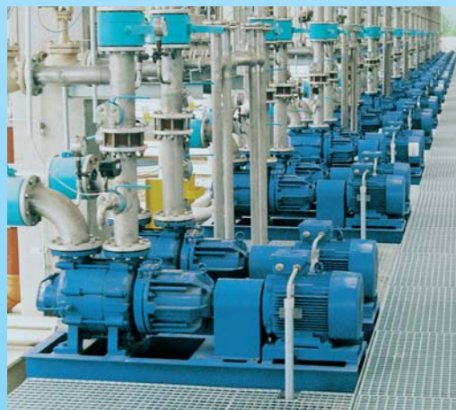
Type HZSM with magnetic coupling. Liquid: Solvent, 20°C (68°F).
