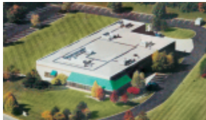
WEST CHESTER, PA FACILITY
