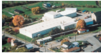
AVONDALE, PA FACILITY
