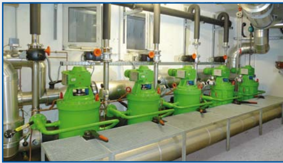
Fig. 3 river water filtration for cooling plant
