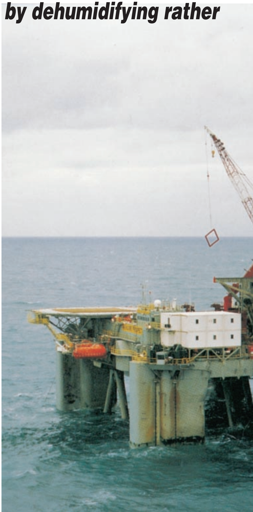
AG dehumidifiers in thruster rooms and lifeboats increase safety and reduce the need for maintenance.
