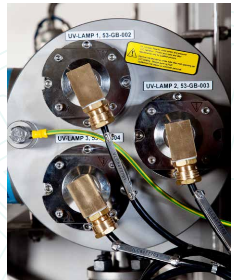
Lamp connection in Ex-safe and service-friendly construction
